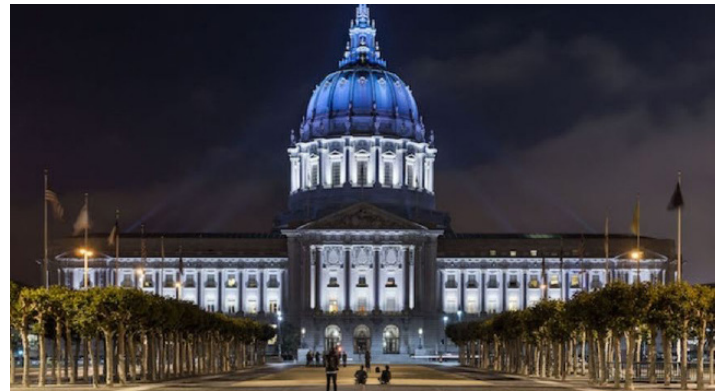
Civic Center Plaza Repair San Francisco Public Works
