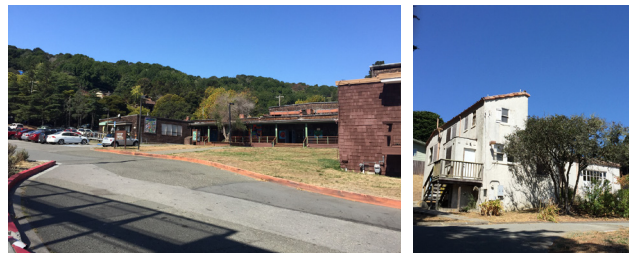
Figure 4: Existing Main Building – Manzanita Recreation Center
